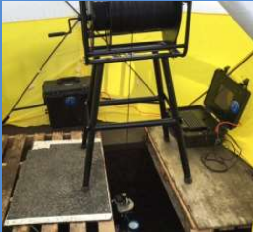
Cable insertion into live water pipe
