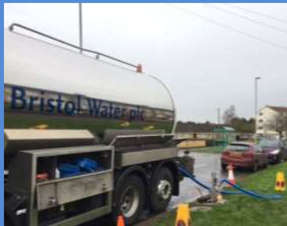
Water tanker flushing prior to CCTV survey
