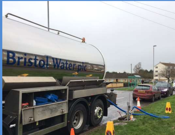
Back feeding water using water tanker
